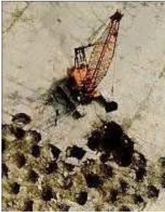
Figure 8-2 – Compactage dynamique
