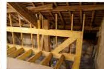
Structure poteau/poutre treillis
