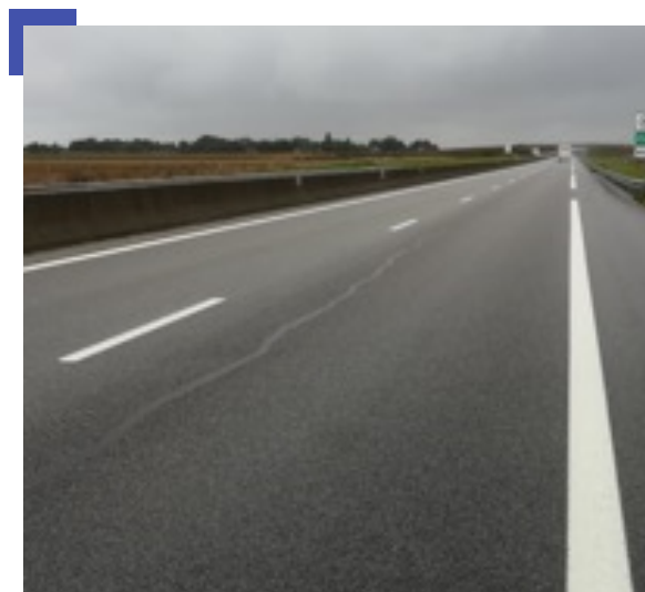
Autoroute A28, Sens 1, PR 250, 02/10/19, BV
