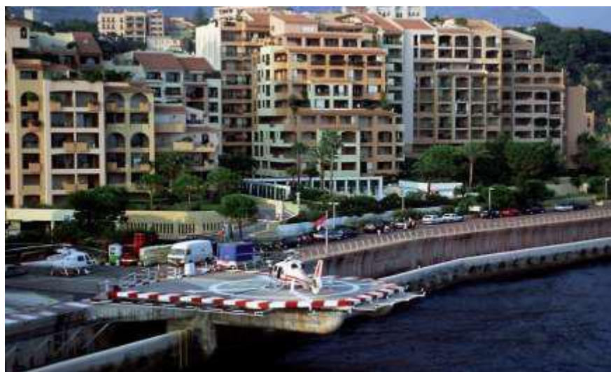
Aerial view of the Monaco heliport, the final approach and take-off area (FATO) with a Dauphin (© Alexandre PARINGAUX / DGAC – STAC)
