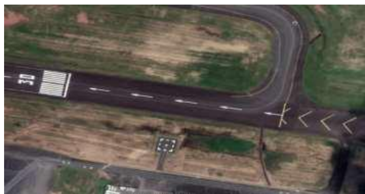
Pointe-à-Pitre Le Raizet Airport (PTP), FATO close to runway, threshold 30 (source: Google Earth)
