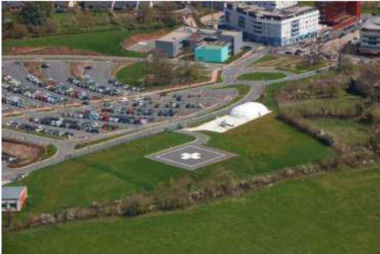
Aerial view of the Rodez helipad (France): Final Approach and Take-off Area (FATO) (STAC: © Photo from STAC / Christian BOUSQUET)
